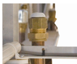
Figure 3.13 Vacuum Breaker
